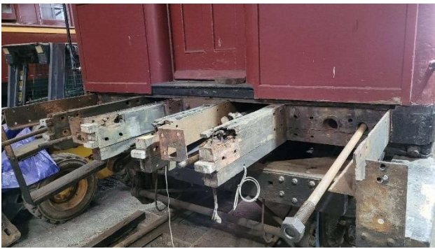
As found upon dismantling the end section.
