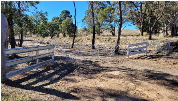
Fencing installed at Hazelgrove.
